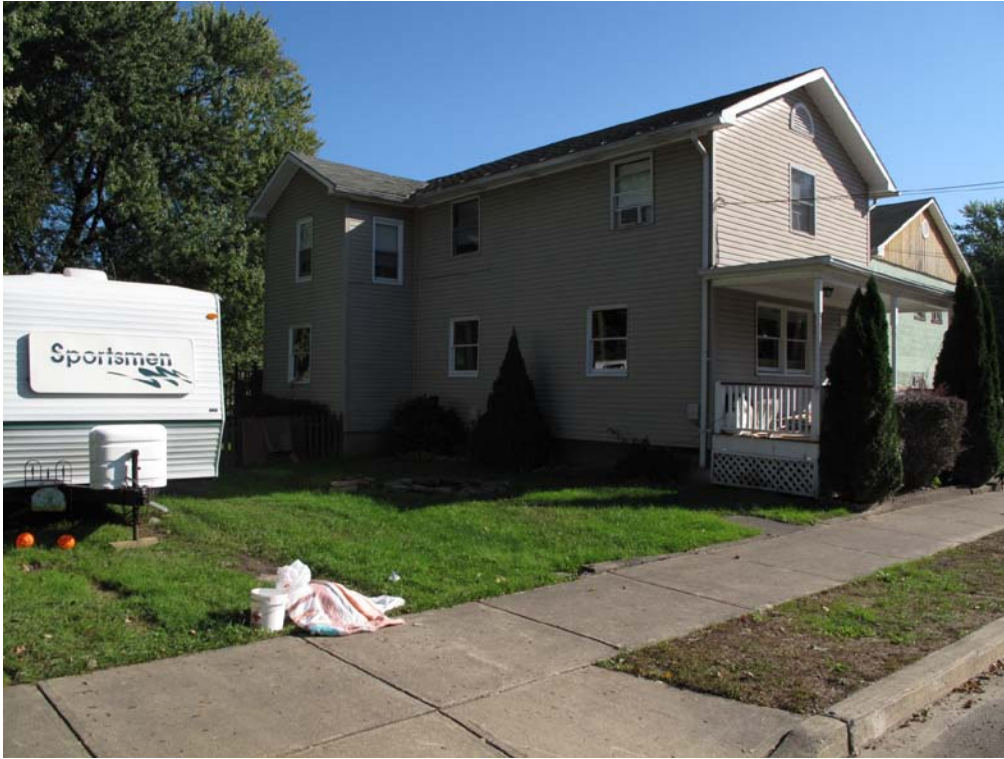
Photo 3 – View of west elevation. Photo looking east.
