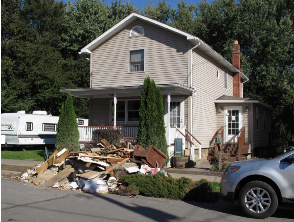
Photo 1 – View of south and east elevations. Photo looking north.
