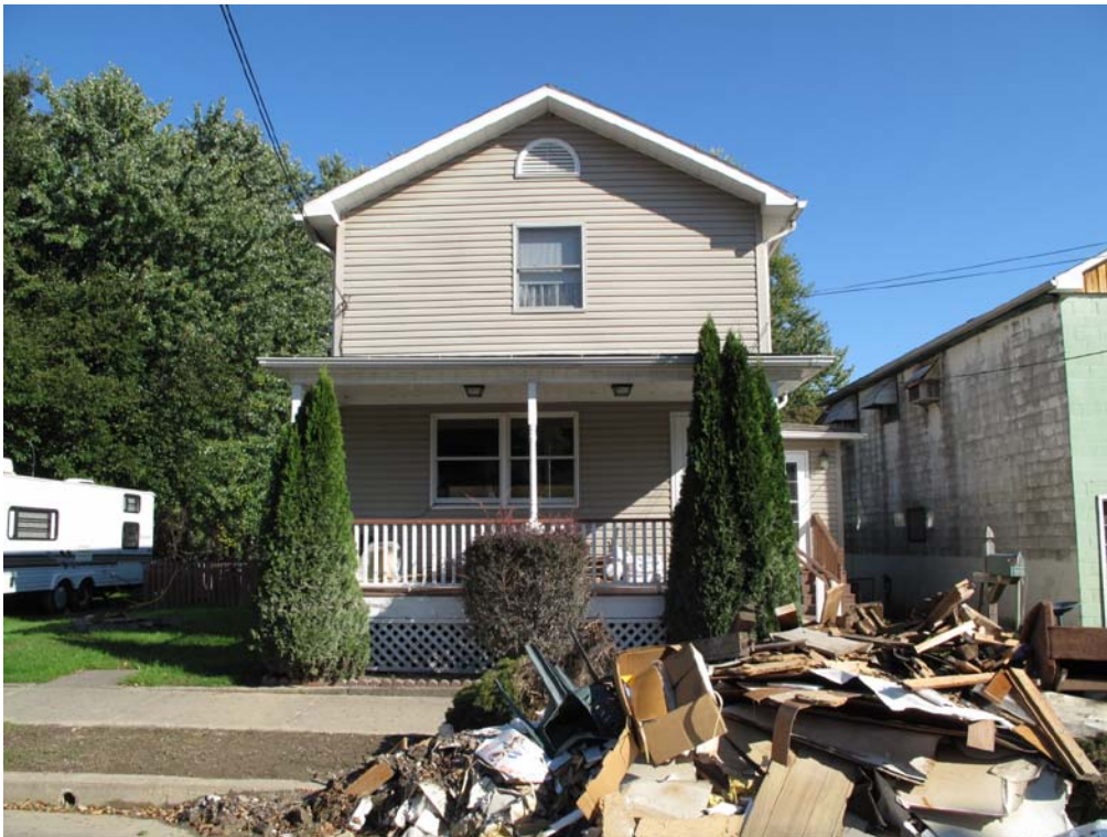
Photo 2 – View of front (south elevation). Photo looking north.
