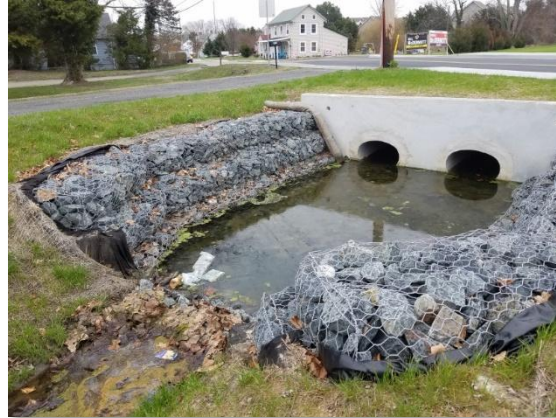
Localized Flood Risk Reduction (Culvert Improvement)
