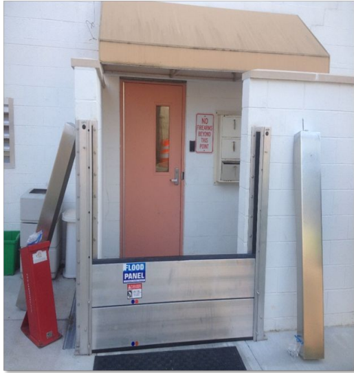
Dry Floodproofing: Non-Residential Structures
